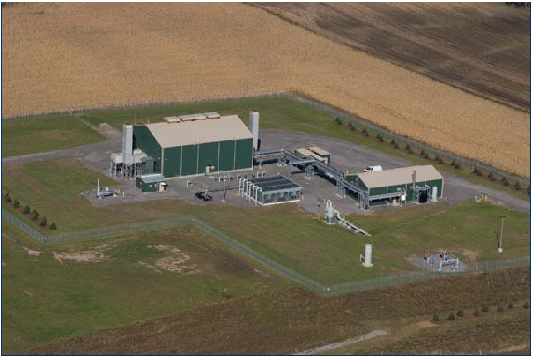
Oakfield, NY Compressor Station
